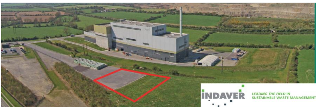
Figure 9: Current view of Meath plant with proposed hydrogen facility location outlined.
