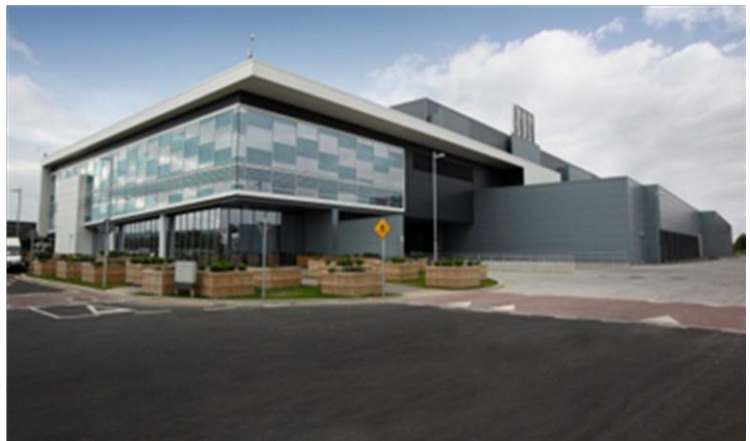
Microsoft's Dublin data centre, an important development for next-generation innovations in Cloud Computing.
